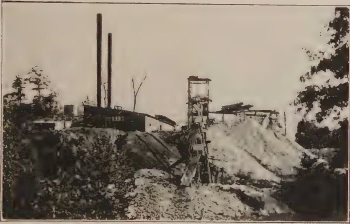
(14) Surface plant at main shaft of Mary Belle mine.
